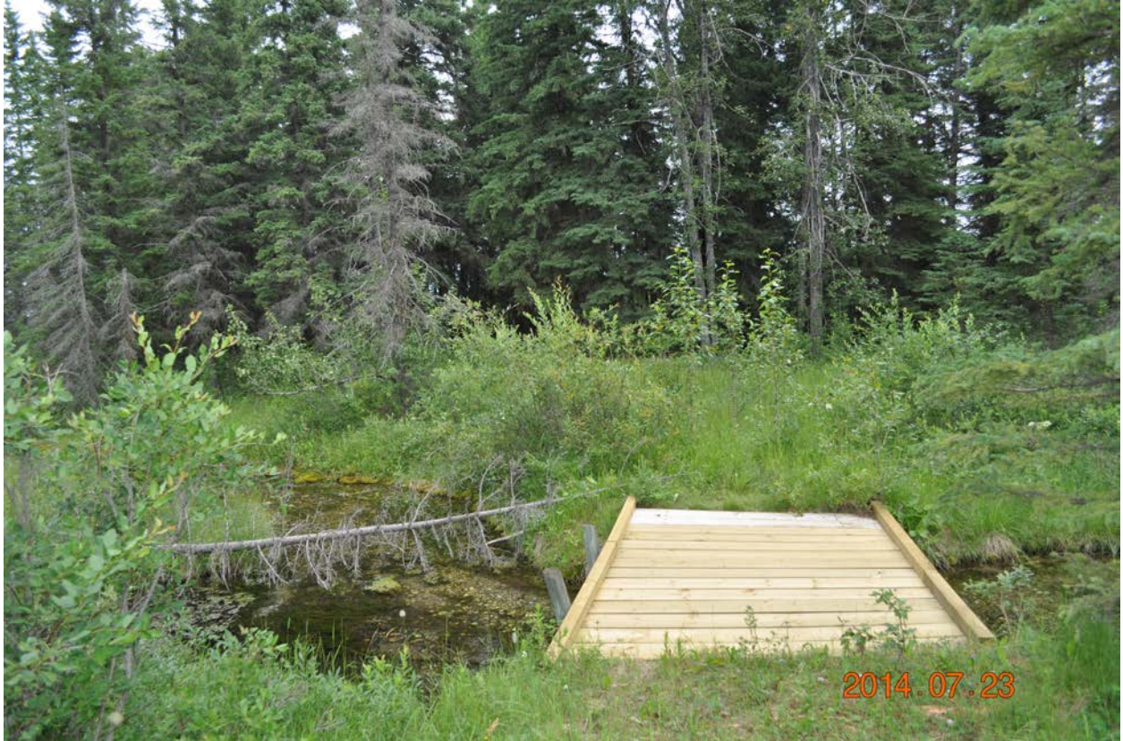
Repaired footbridge at Stainbrook Springs Conservation Site. Photo: Mandy Couve
