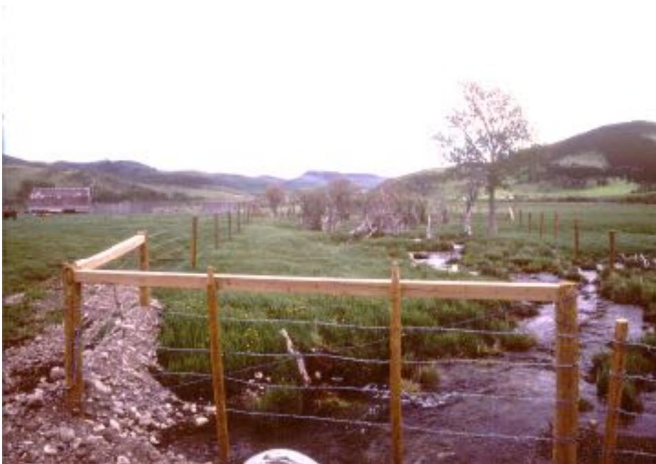
Goat Creek (Todd Creek Tributary) after initial installation of Streambank Fencing (1993).
