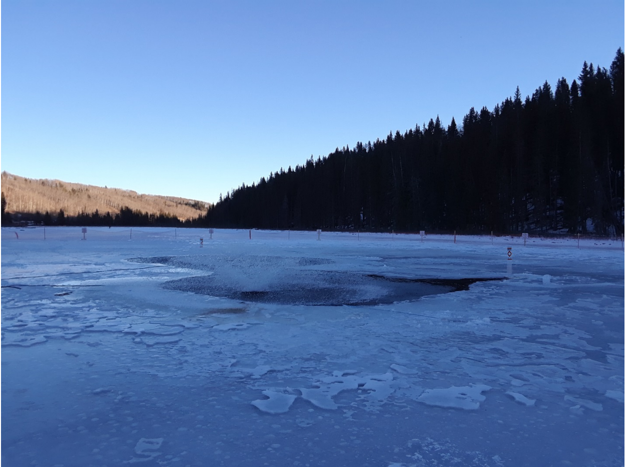
Fountain action of the surface aerators shortly after being powered on for the first time at Winchell Lake. Photo: Andrew Clough
