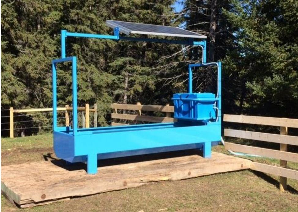
A solar-powered off-site watering system installed to prevent cattle access to the Raven River.
