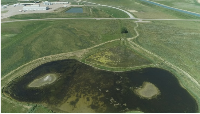
Photo 3. Drone imagery of the constructed wetland on the west end of Ridge Reservoir. Photo: Jeff Forsyth
