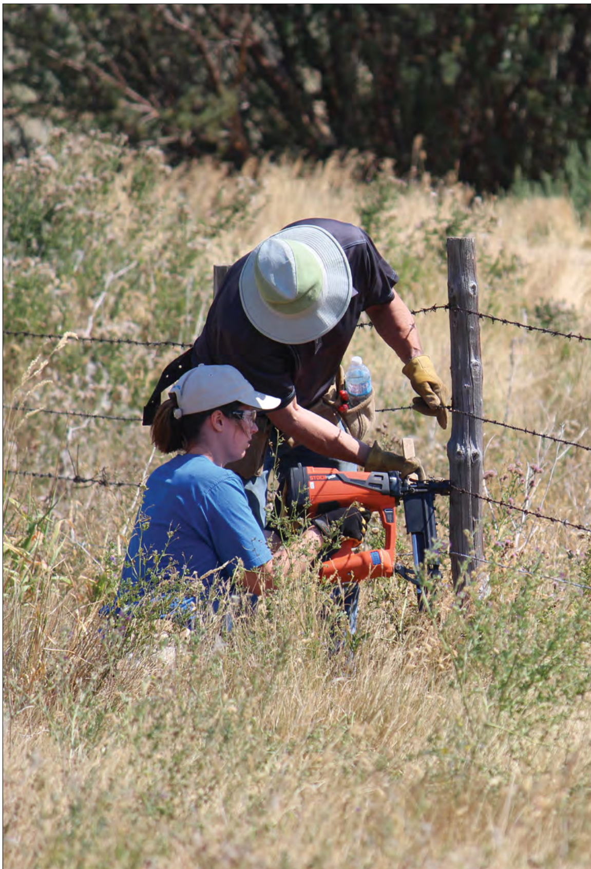
Securing smooth wire 46 cm off the ground photo: ACA, Mike Verhage
