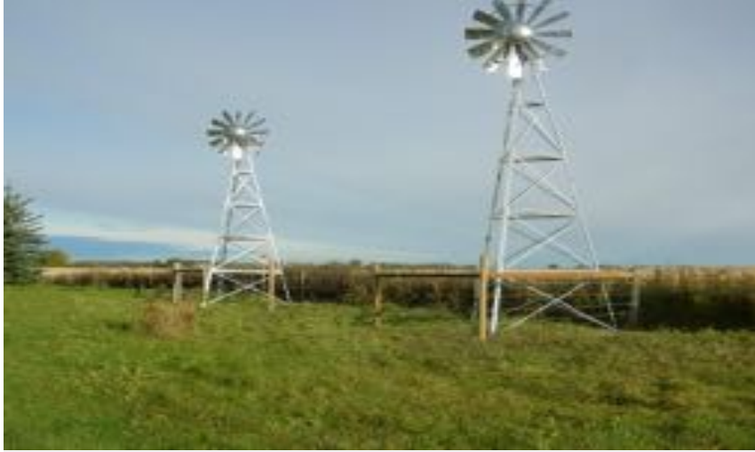
Six meter windmill aerators at Boehlke Pond. (Photo: Diana Rung)
