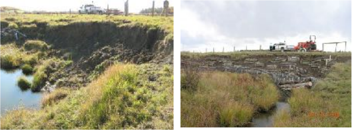
Figure 4. Before (left) and after (right) photos of the bank stabilization project completed in 2008 (Photographs by Kelly Hooey).
