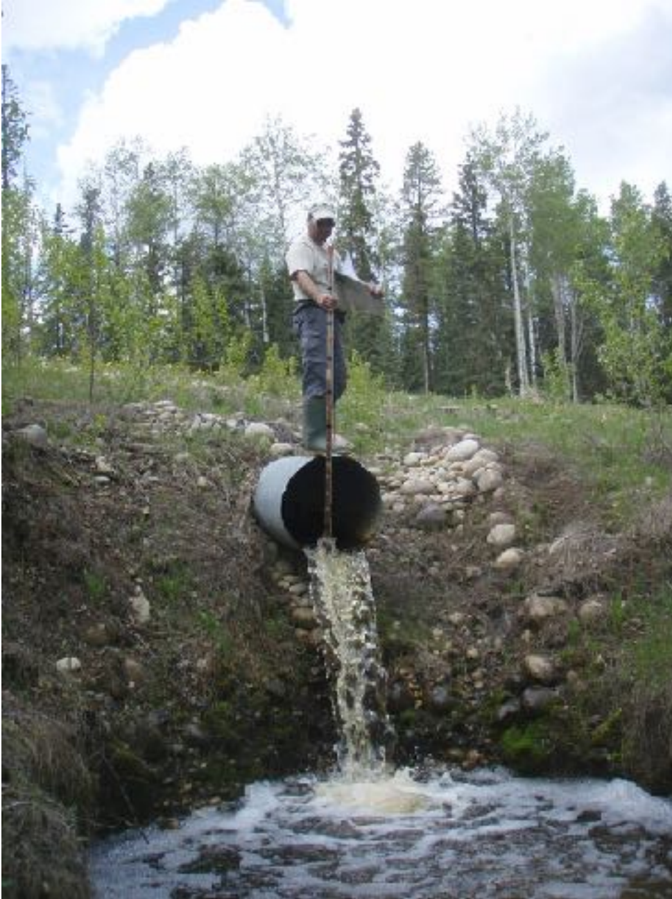
Photo 2. Hanging culvert in the Sakwatamau River drainage. Photocredit Laura MacPherson
