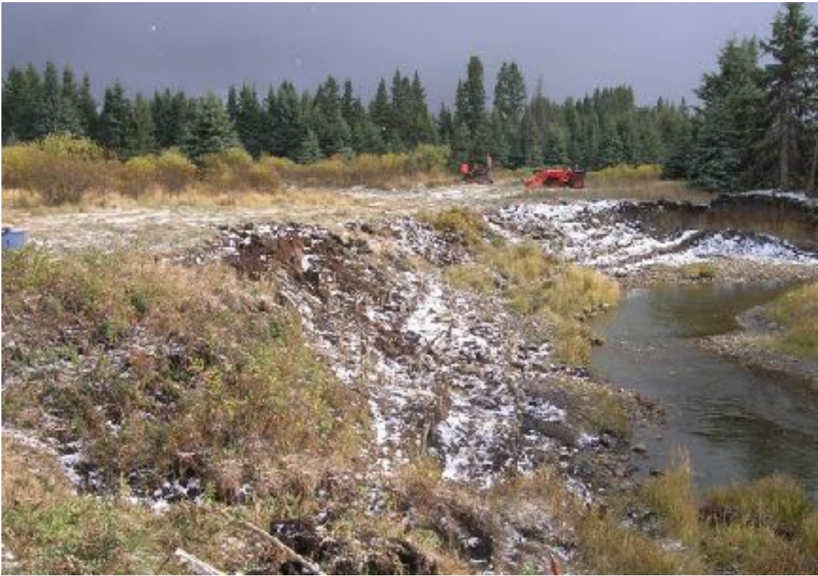
Bank stabilization project using bioengineering at site ACAB09-3 located on NW-11-33-06-W5. (Photo: Kelly Hooey)
