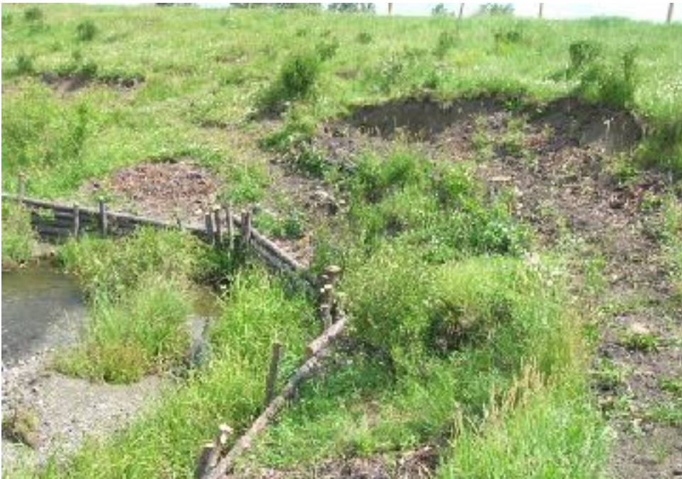
Bank stabilization project using bioengineering at site ACAB09-1 located on NE-17-33-07-W5. (Photo: Kelly Hooey)
