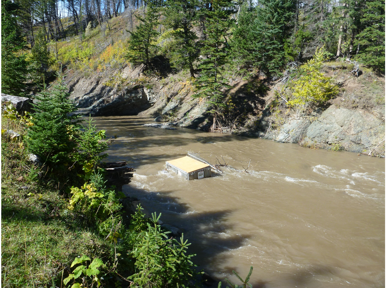
Conduit fish trap in the Carbondale River failed because of high stream flows. Photo: Leah Neigum
