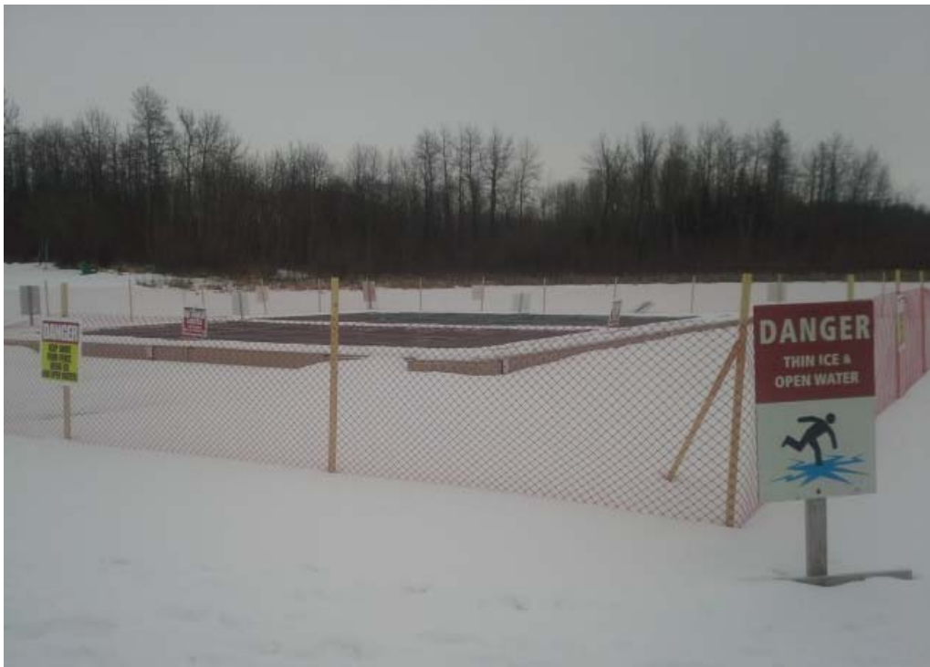
Thin ice warning signs and high visibility perimeter fencing installed around PolyDock structure at Muir Lake. Photo: Troy Furukawa
