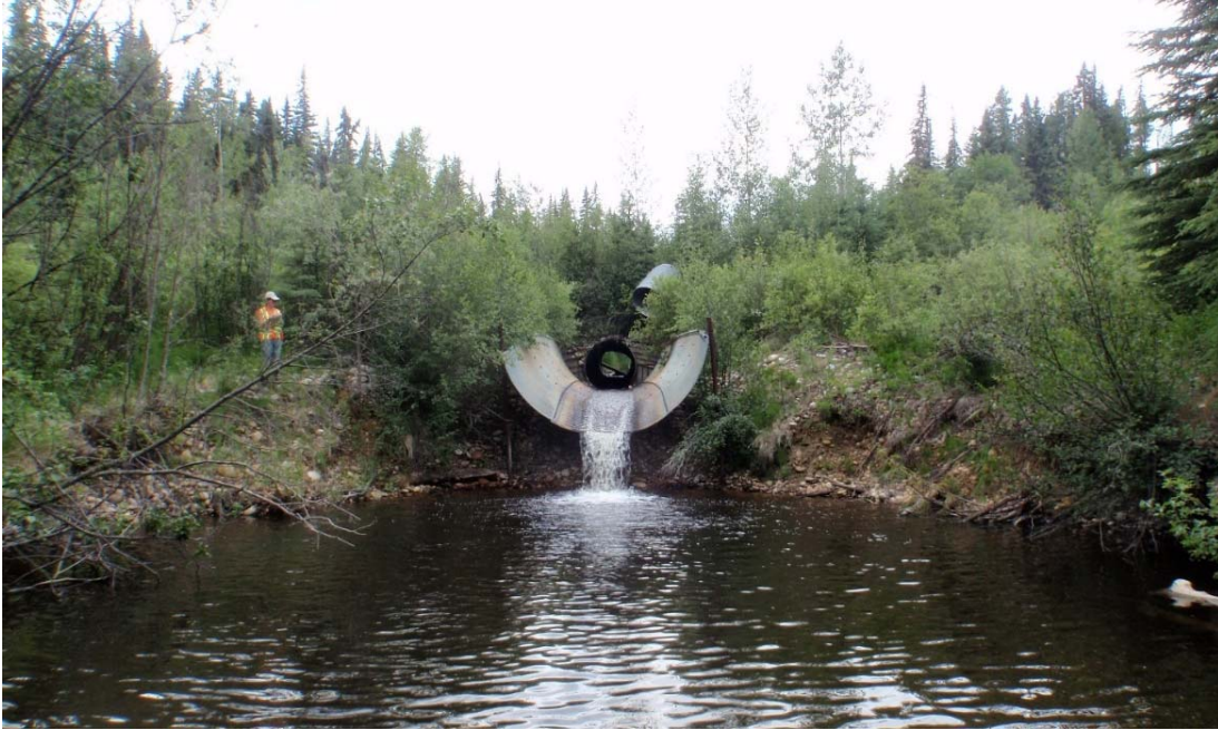
An example of one of many perched culverts that fragment fish habitat in the Swan River watershed. Photo: Troy Furukawa
