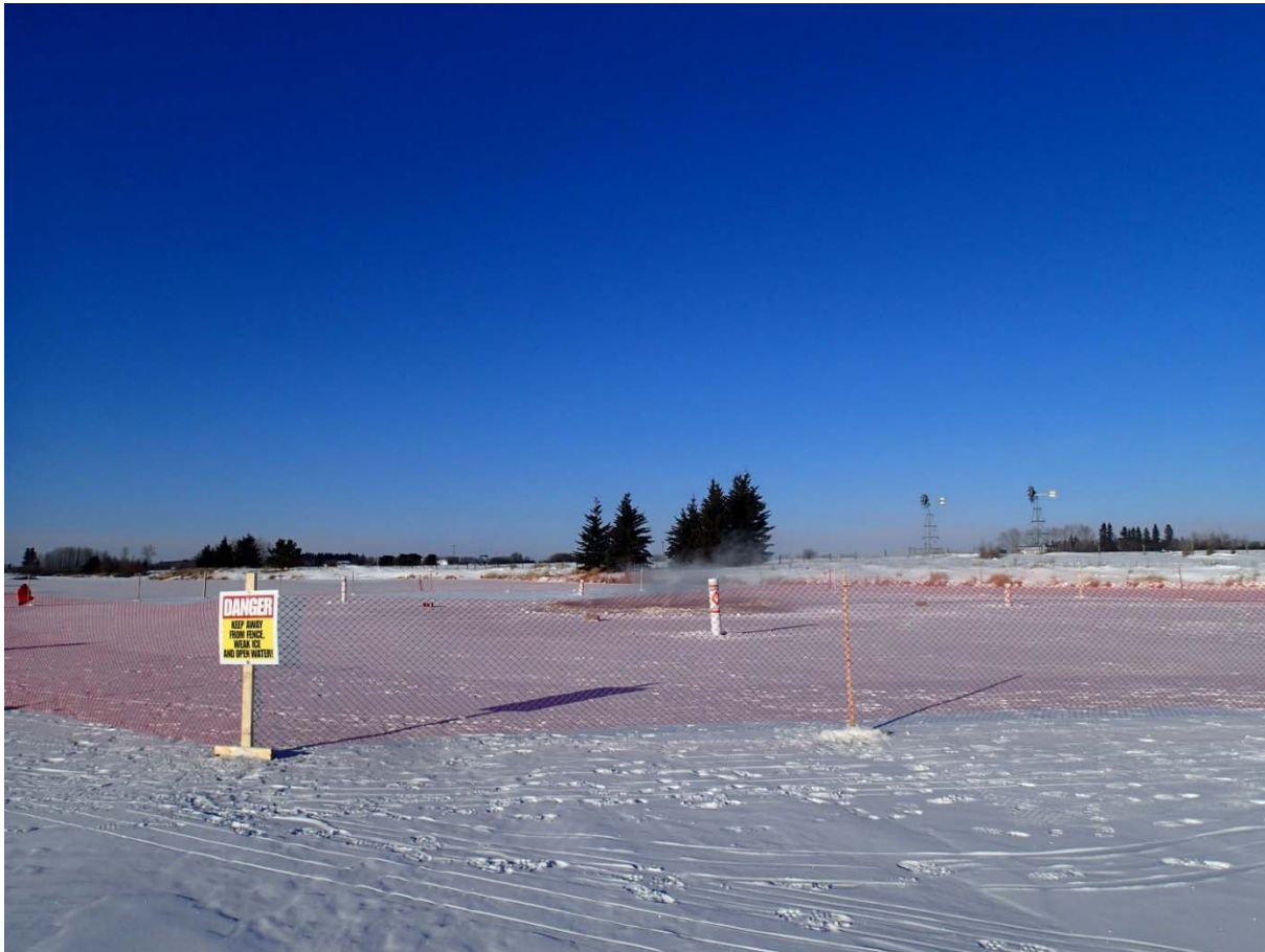
Operation of surface aerators at Hansen's Reservoir. Photo: Chad Judd
