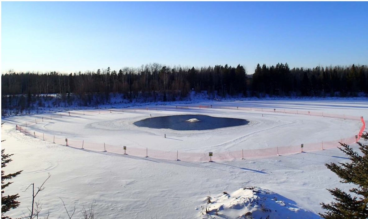
Mechanical surface aerator and perimeter fence installed at Ironside Pond. Photo: Chad Judd
