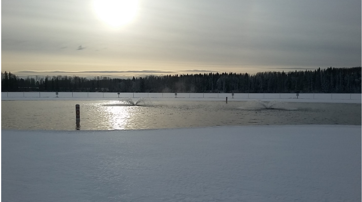
Surface aerators with perimeter fence in background at Spring Lake (Stony Plain). Photo: Brendan Ganton
