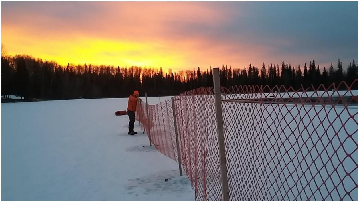
ACA staff installing perimeter fence at Millers Lake. Photo: Brendan Ganton
