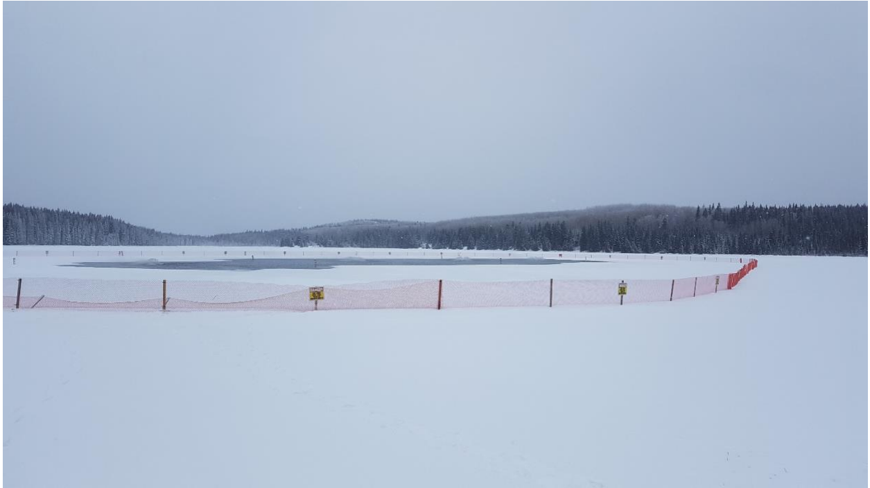
Surface aerators with perimeter fence at Sulphur Lake. Photo: Nikita Lebedynski
