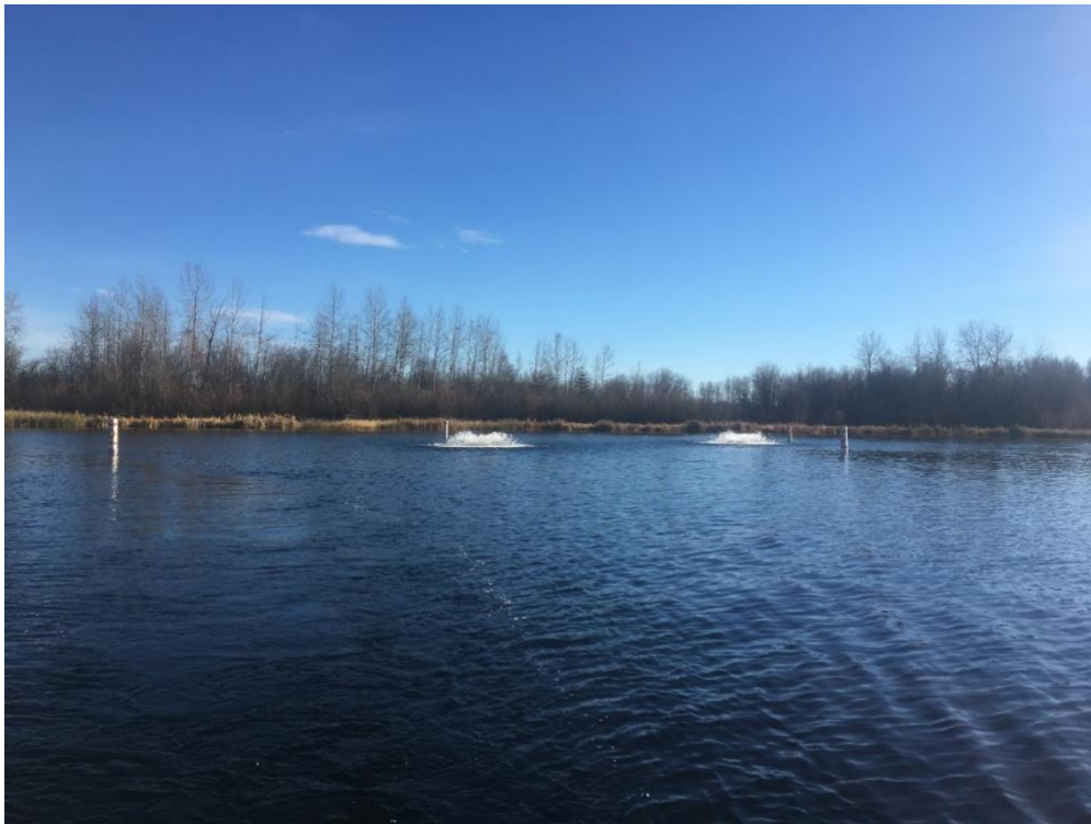
Fountain action of surface aerators shortly after being powered on for the first time at West Dollar Lake. Photo: Scott Seward
