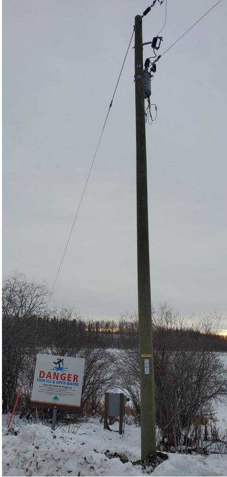
Photo 2. Newly installed power line at Peanut Lake. Photo: Troy Furukawa
