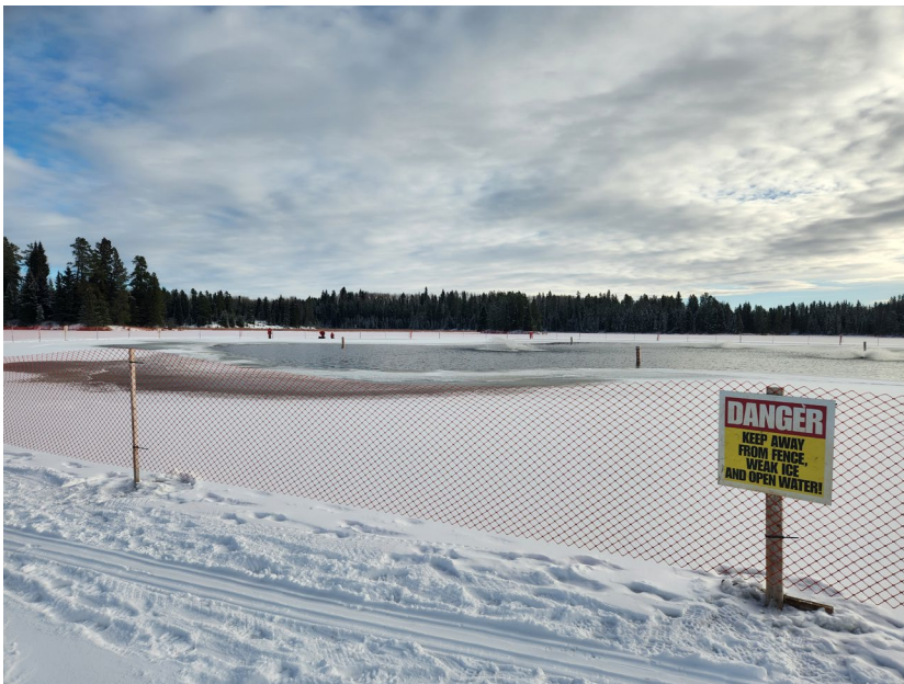
Photo 2. Safety fence and signage installation at Beaver Lake. Photo: Andrew Clough
