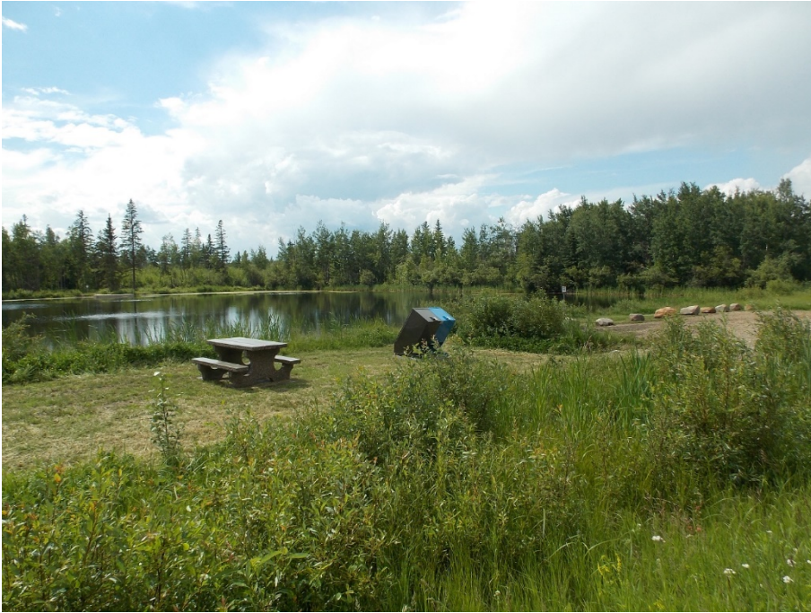
Photo 1. Diffuser aeration at Shell True North Pond. Photo: Garret Mcken
