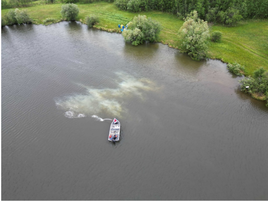
Photo 3. Aerial photo of aluminum sulphate being applied to Westlock Pond using a pump, discharge hose, and boat. Photo: Northern Lights Fly Fishers
