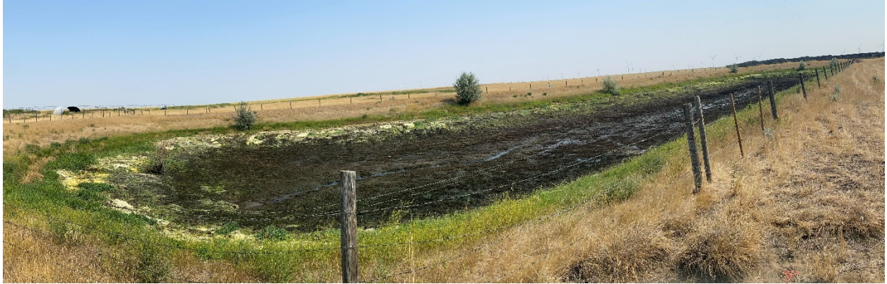
Photo 3. Partially decomposed vegetation that remained in the pond basin after draining. Photo: Brad Hurkett
