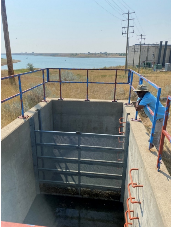
Photo 5. Alberta Conservation Association Fisheries Resource Program Manager observing pond water draining through the fish harvest kettle before flowing back into Forty Mile Coulee Reservoir. Photo: Brad Hurkett
