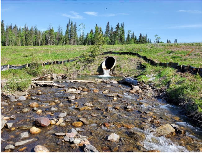
Photo 1. A barrier to upstream fish movement that is being remediated. Photo: Chad Judd.
