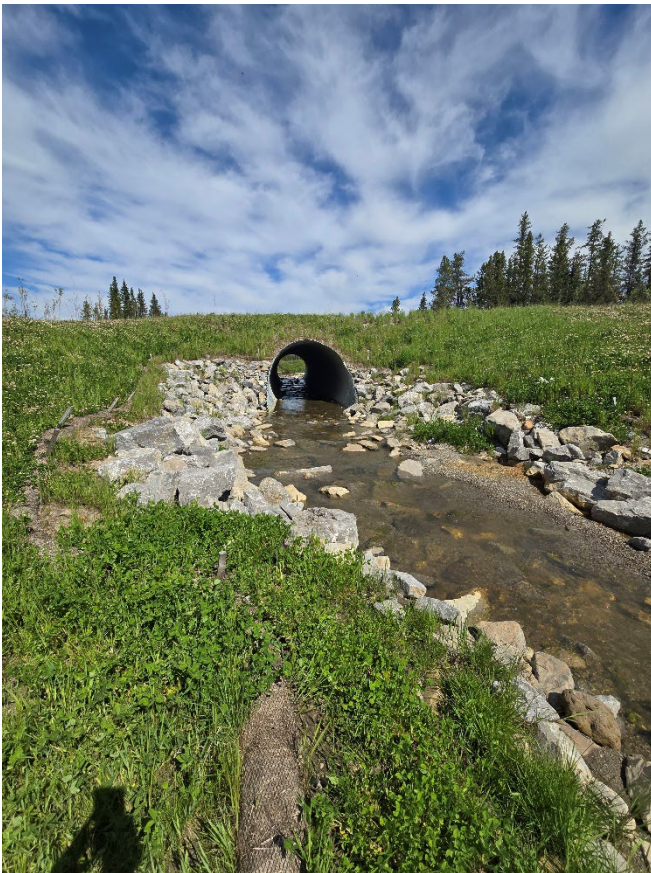
Photo 2. A recently remediated crossing that was assessed in 2024. Photo: Chad Judd
