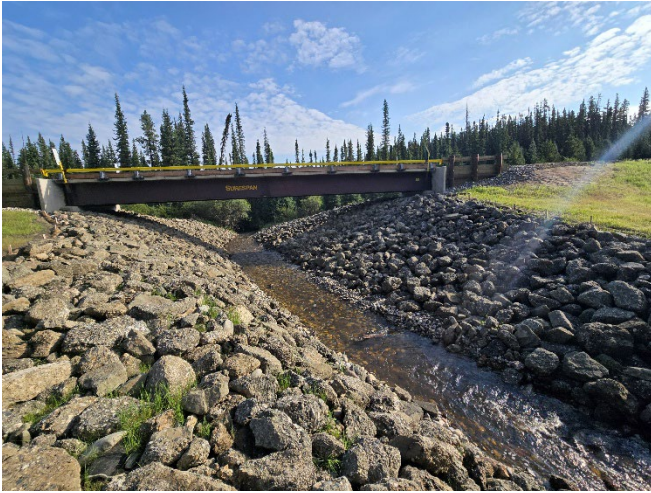
Photo 1. A newly constructed bridge crossing over Deerlick Creek, McLeod River watershed. Photo: Chad Judd
