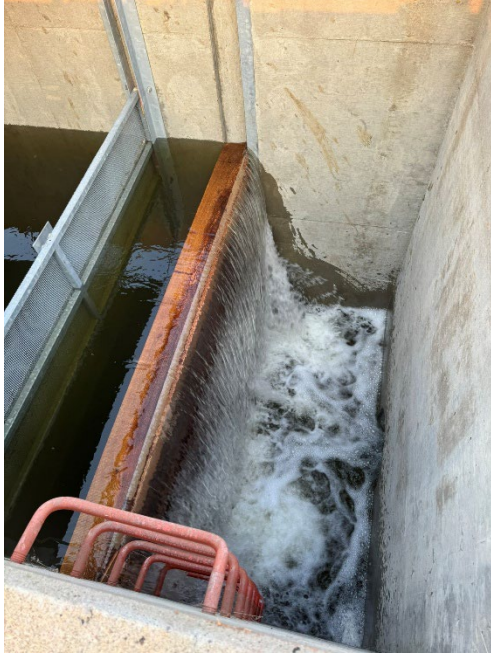
Photo 3. Water draining over drop boards in the fish extraction kettle at the Forty Mile walleye rearing pond. Photo: Brad Hurkett
