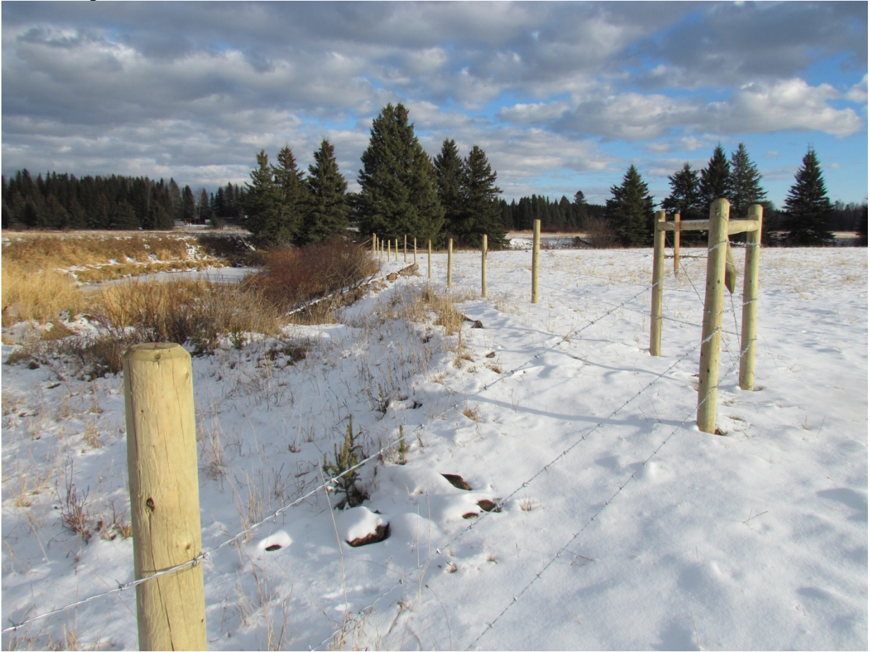
A portion of new wildlife-friendly livestock exclusion fence installed on the Edson River. Photo: Juanna Thompson [Photo1_Riparian Edson_2013-14_Juanna Thompson.jpg]
