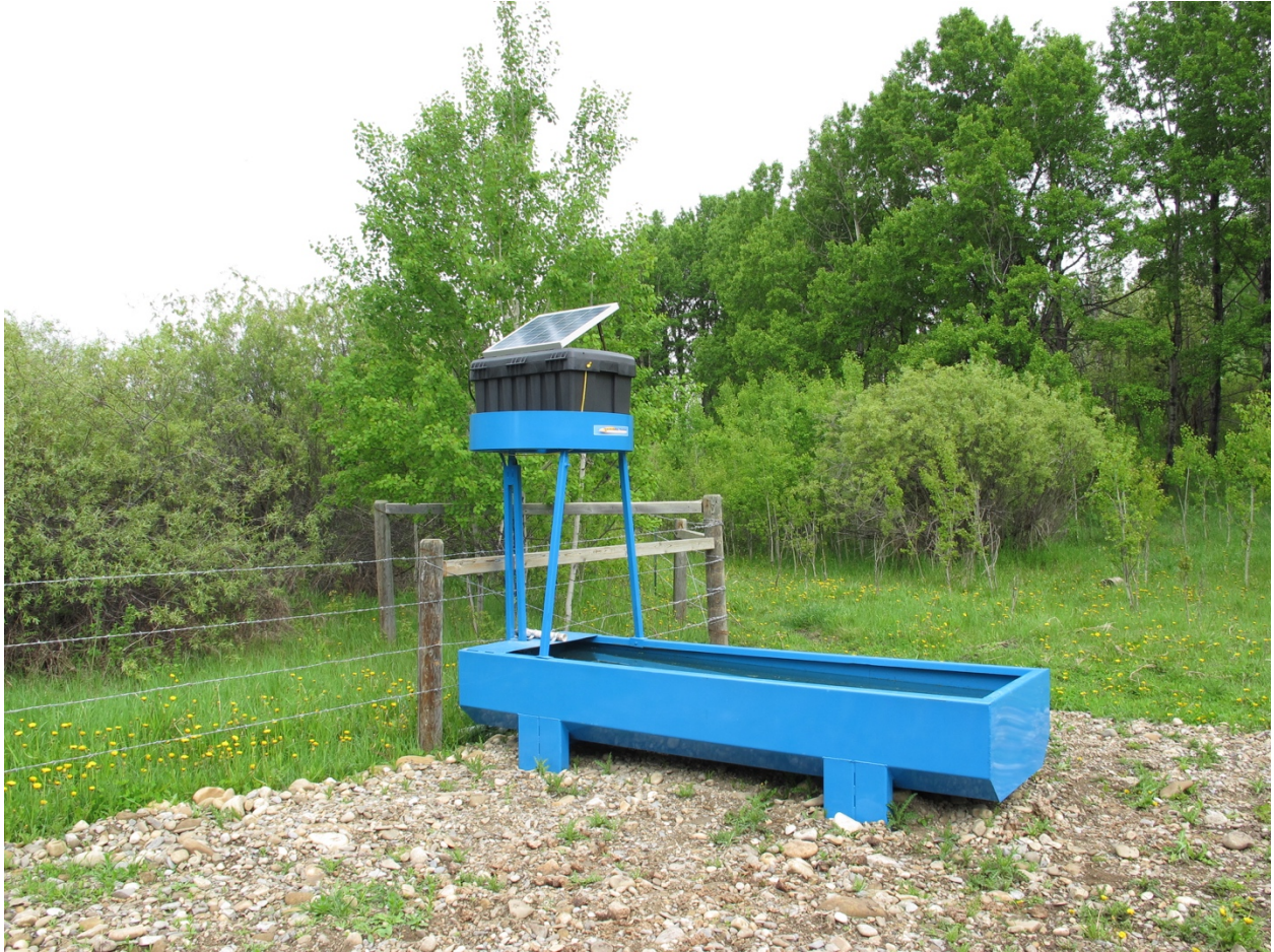
Off-site watering system installed to protect riparian habitat. Photo: Erin VanderMarel [Photo2_Riparian NRR_2013-14_Erin VanderMarel.jpg]
