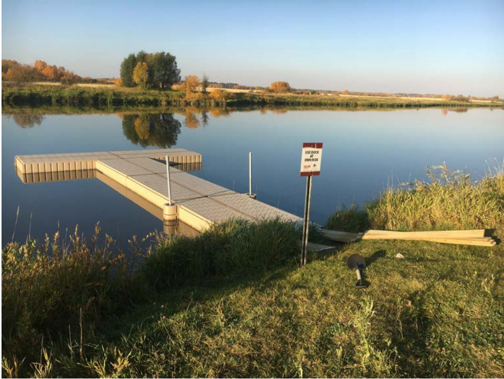
New floating dock installed at Hansen's Reservoir. Photo: Marco Fontana
