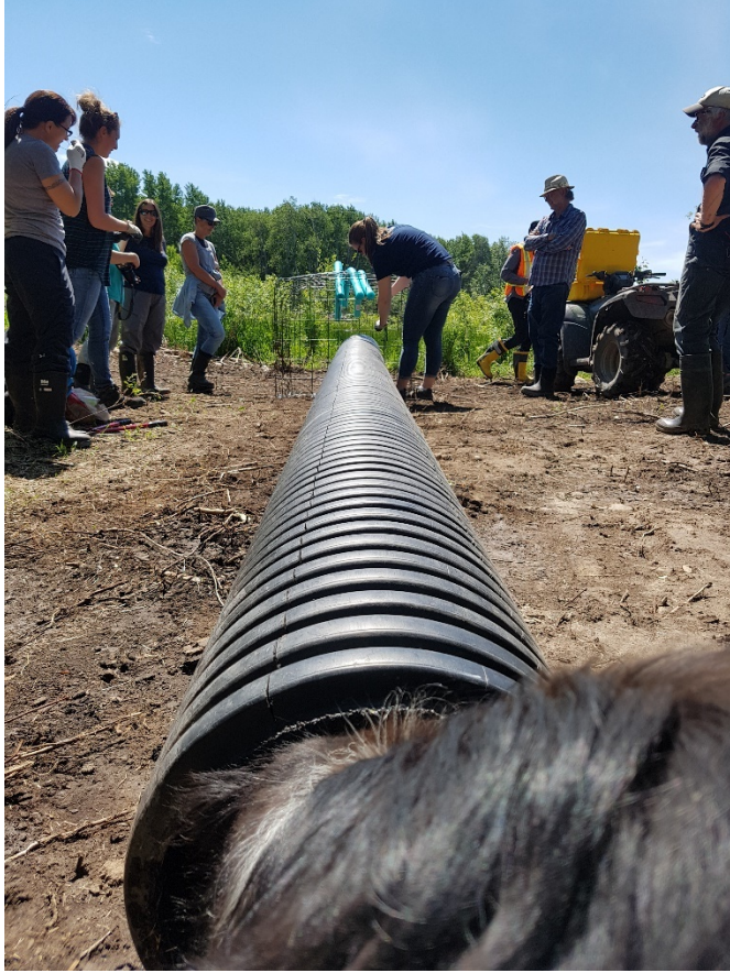
Pond leveler installation on Windsor Creek with participating landowner. Photo: Garret McKen
