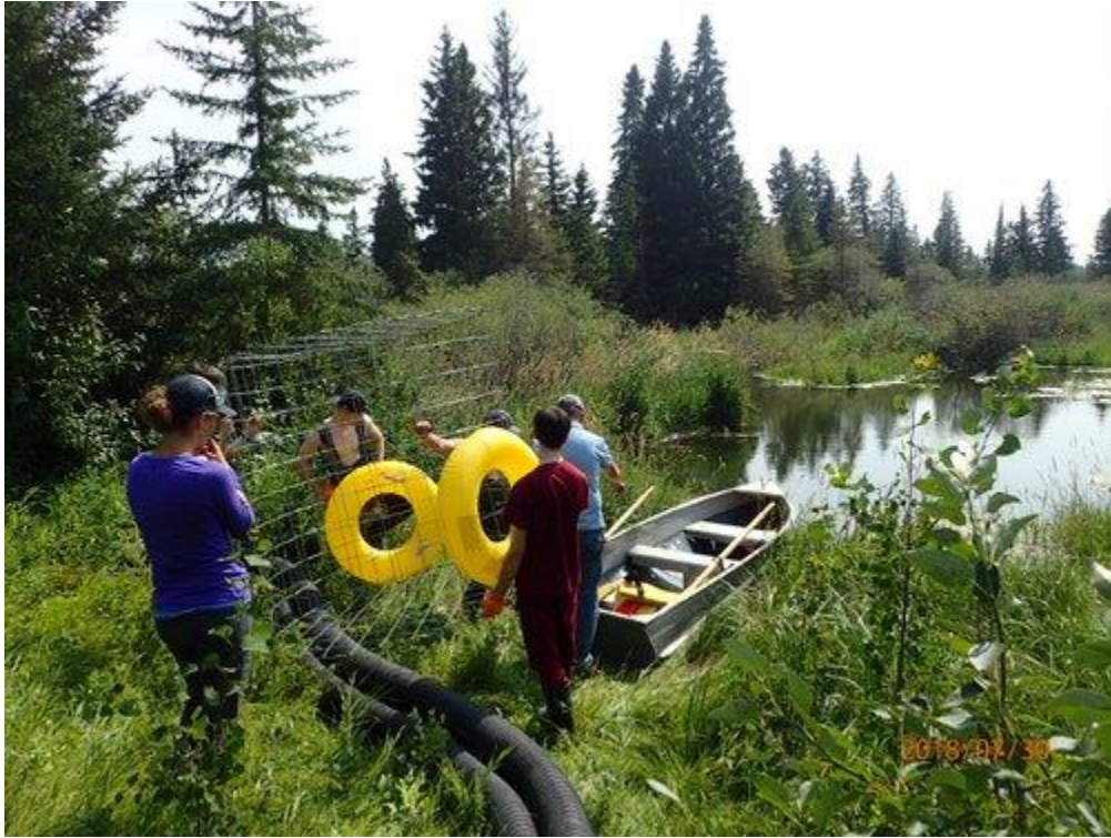
Beaver pond leveler installation at Porter Conservation Site. Photo: Mandy Couve
