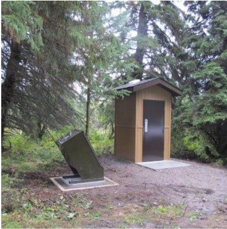
A new outhouse and bearproof garbage can installed at Coulson Conservation Site. Photo: Marco Fontana
