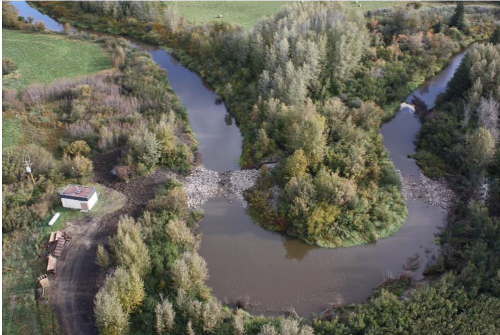
Aerial image of the Beaverlodge River at the weir with the two natural rock passage structures. These structures change the gradient of the river so that fish can pass over the weir in times of low flows. Photo: Nikita Lebedynski
