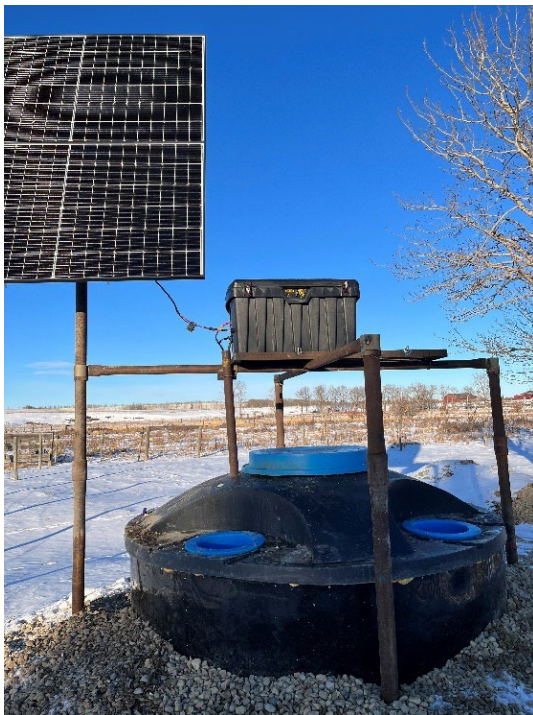
Photo 2. New solar off-site watering unit installed on Dogpound Creek.
