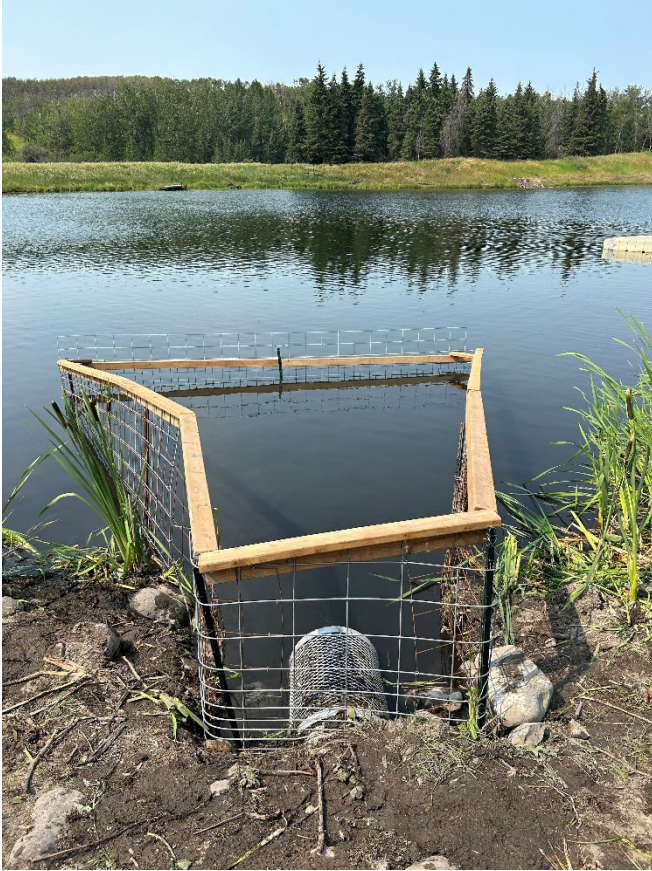
Photo 1. Beaver exclusion fence constructed at the outflow of Boulder Lake Conservation Site. Photo: Diana Rung
