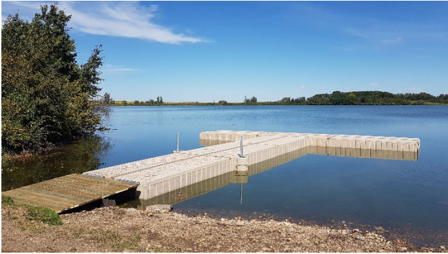
Photo 1. Floating dock installed at Windsor Lake. Photo: ACA
