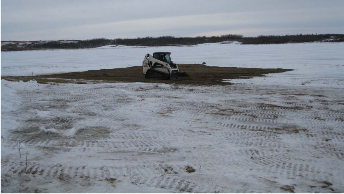
We spread the gravel with a bobcat in the winter, and then we made some fine-scale adjustments in the spring by hand to create piping plover breeding habitat along the shoreline of a waterbody at Junction Lake Conservation Site. Photo: Amanda Rezansoff
