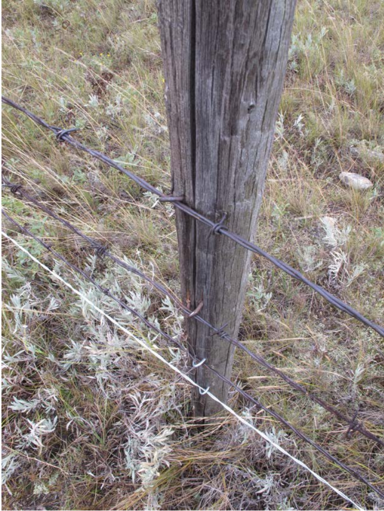
An image of a barbed-wire fence where the bottom strand has been replaced with double-stranded smooth wire and its height adjusted to 46 centimetres. Photo: Robert Anderson
