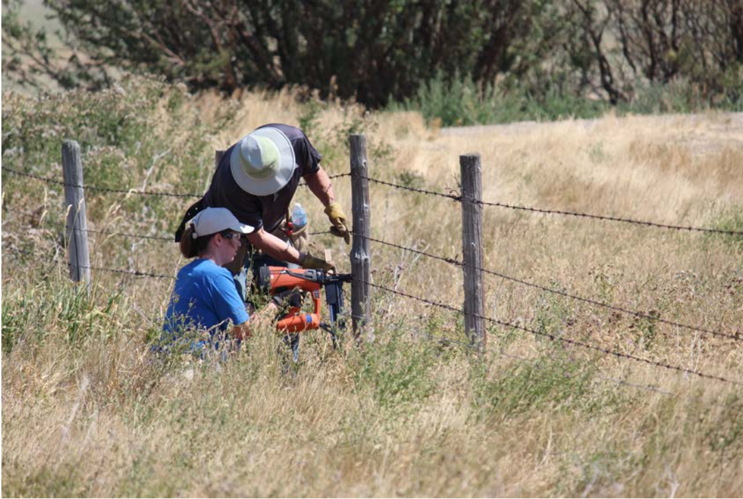
Alberta Conservation Association staff member Jennifer Baker and a volunteer secure the bottom smooth wire at 46 centimetres above ground with a power stapler. Photo: Mike Verhage
