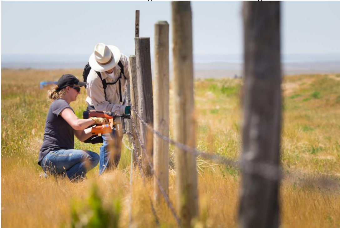
ACA staff member, Amanda MacDonald, and Alberta Fish & Game Association volunteer use a power stapler to respace existing barbed wires and secure the bottom smooth wire at 46 cm (roughly knee height) above ground. Photo: Jason Headley
