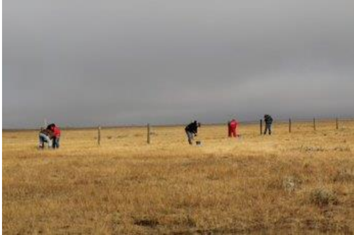
Alberta Fish & Game Association volunteers enhancing a barbed-wire fence by securing the bottom smooth wire at 46 cm above ground. Photo: Mike Verhage
