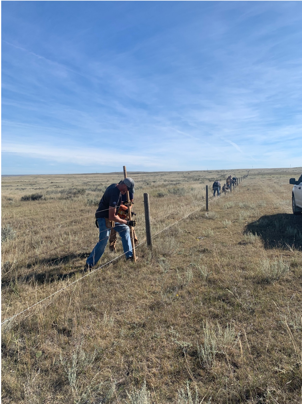
ACA staff member, Mike Verhage, and AFGA volunteer use a measuring stick to space wires at recommended distances as a power stapler is used to secure the wires, with the bottom smooth wire at 46 cm (roughly knee height) above ground. Photo: Amanda MacDonald
