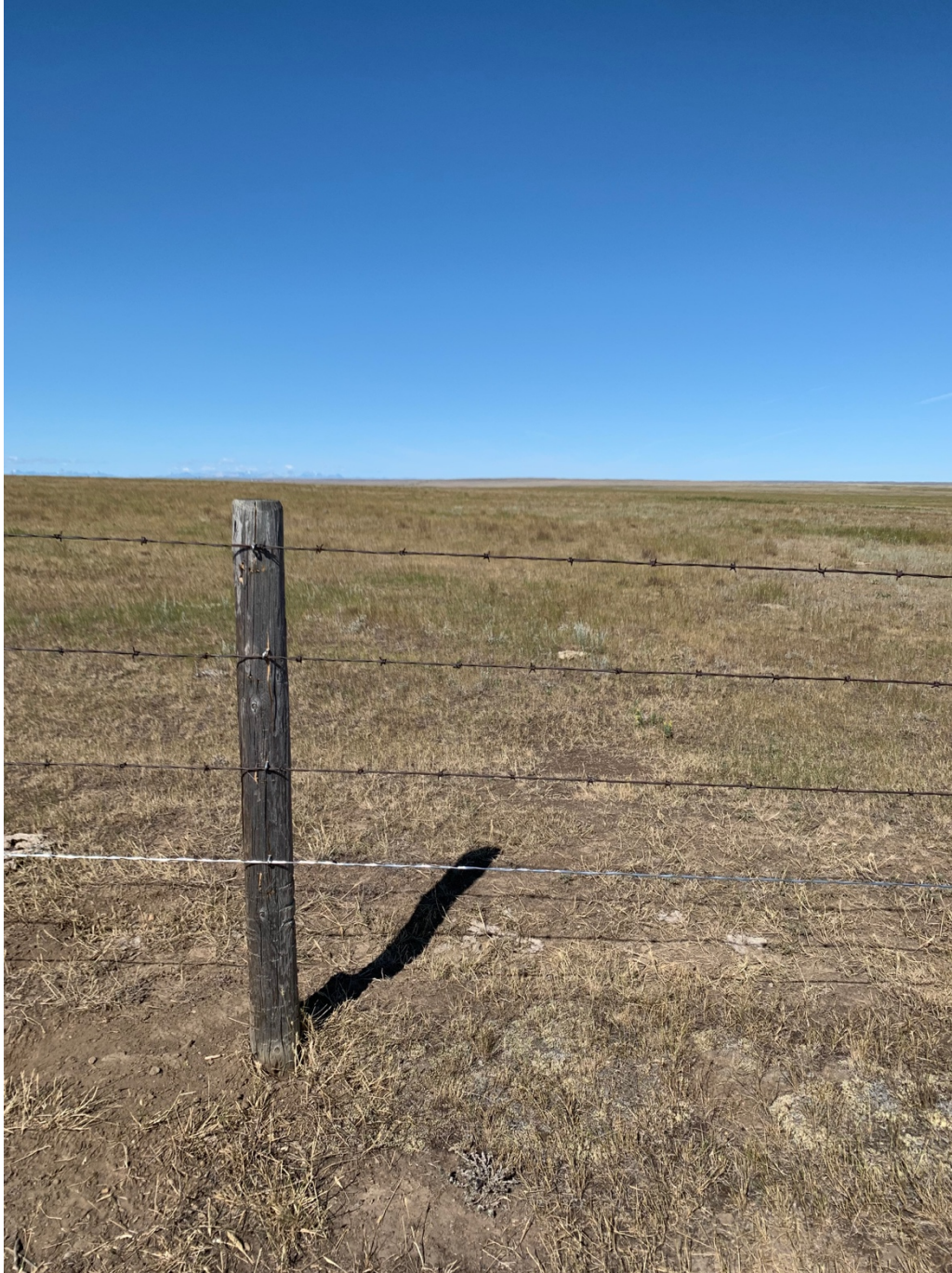
Completed section of modified fence with the bottom strand of barbed wire removed and replaced with smooth wire secured at 46 cm (roughly knee height) above ground and remaining strands of barbed wire re-spaced to equal intervals. Photo: Amanda MacDonald
