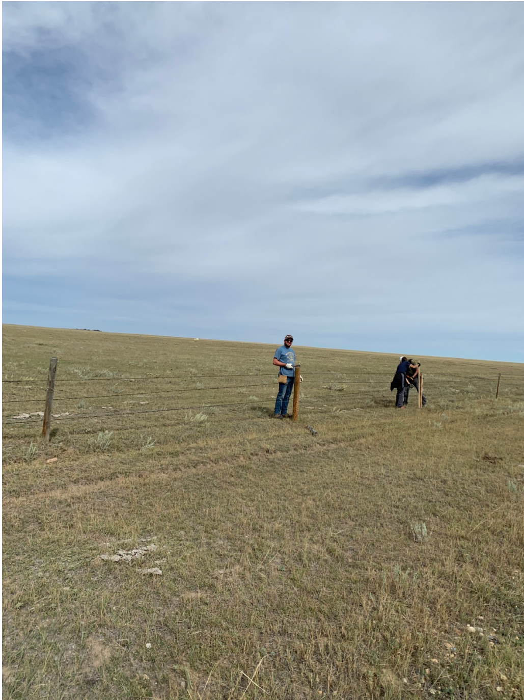
ACA staff member, Scott Vegter, preparing existing barbed wire strands to be re-spaced by pulling fencing staples while volunteers use a power stapler to secure the wires, with the bottom smooth wire at 46 cm (roughly knee height) above the ground and remaining strands secured at equal intervals. Photo: Amanda MacDonald
