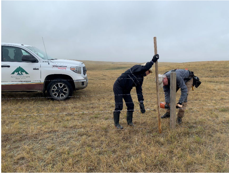
Photo 1. AFGA volunteers using a measuring stick to respace the wires and a power stapler to secure them, with the bottom smooth wire set at 46 cm (roughly knee height) above the ground and remaining strands spaced evenly while leaving a 30-cm gap between the top two wires. Photo: Amanda MacDonald
