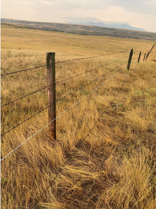
Photo 3. Completed section of modified fence with the bottom strand of barbed wire removed and replaced with smooth wire secured at 46 cm (roughly knee height) above ground and remaining strands of barbed wire respaced evenly. Photo: Amanda MacDonald
