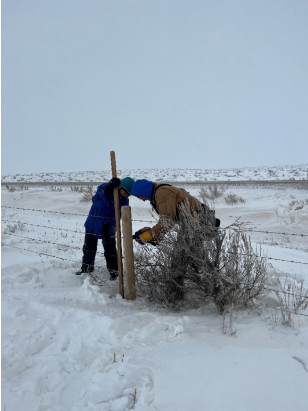
Photo 2. AFGA volunteers working through snow drifts to respace wires with the bottom smooth wire set at 46 cm (roughly knee height) above the ground and remaining strands spaced evenly to 107 cm. Photo: Amanda MacDonald
