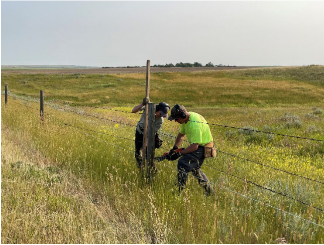
Photo 1. Volunteers modifying an existing fenceline to wildlife-friendlier standards by measuring and securing wires at the appropriate wire heights near Manyberries, AB.
