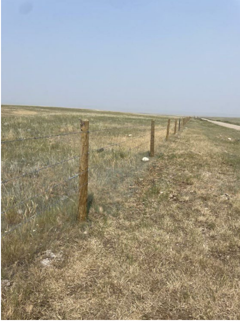
Photo 3. New fenceline installed to wildlife-friendlier standards. Photo: Paige Asplund
