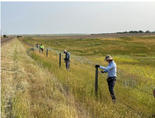
Photo 2. Volunteers removing existing fencing staples in preparation for resecurement at wildlife-friendlier standards near Manyberries, AB. Photo: Tyler Johns
