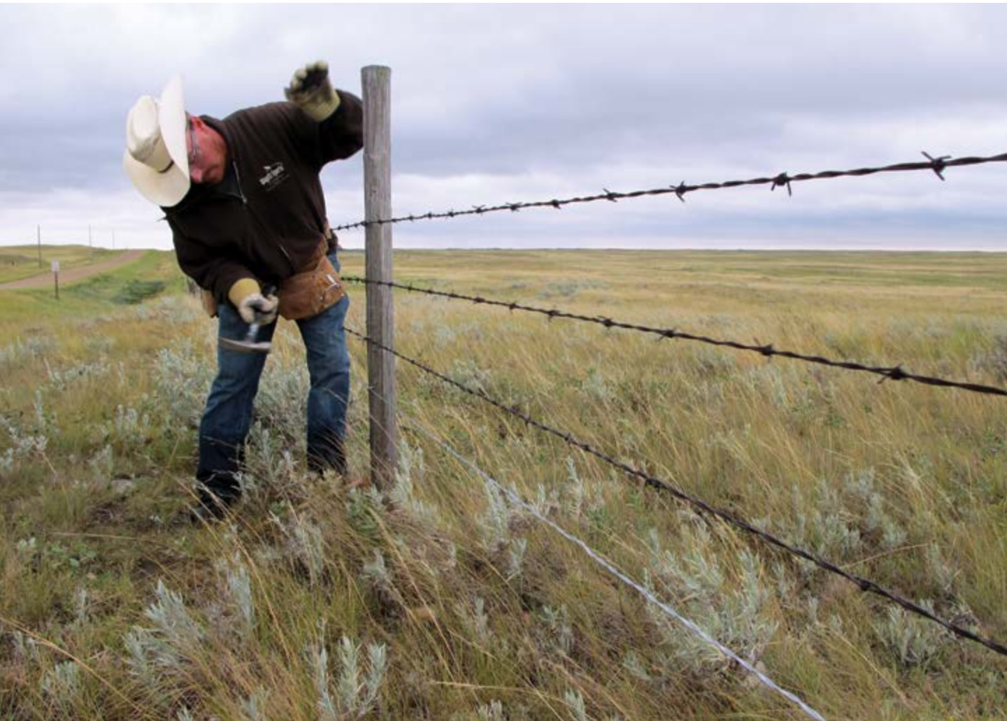
Jeffery Gilham an ACA seasonal employee, staples the bottom double stranded smooth wire making pronghorn passage easier and safer.
